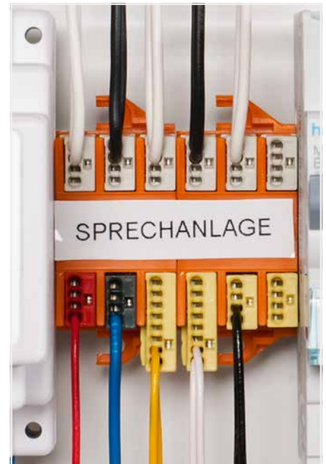
Example of a residential intercom application
