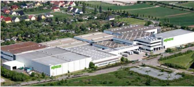
WAGO Sondershausen, Germany
