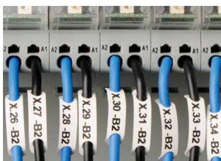
Wire marker for thread-on mounting
